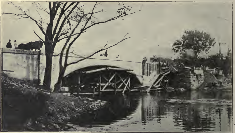
BUILDING THE NEW CONCRETE BRIDGE AT ROME, N. Y.
